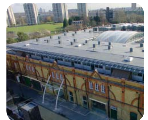
Single floor extension adding 52 additional units
